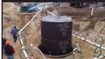
Courthouse Commons Pump Station
